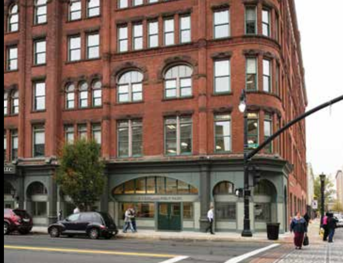
New England Public Radio's beautiful new facilities in a historic Springfield, MA building presented some interesting challenges.
